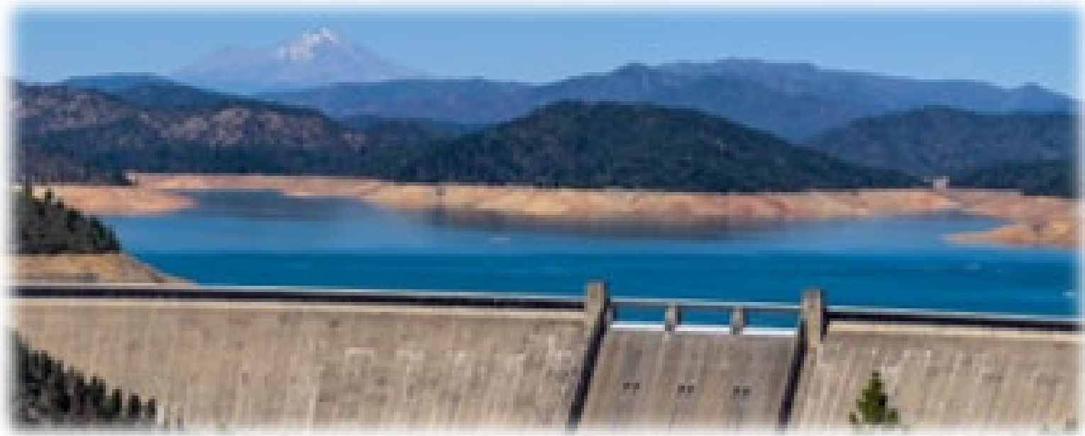
Shasta Dam and Reservoir
