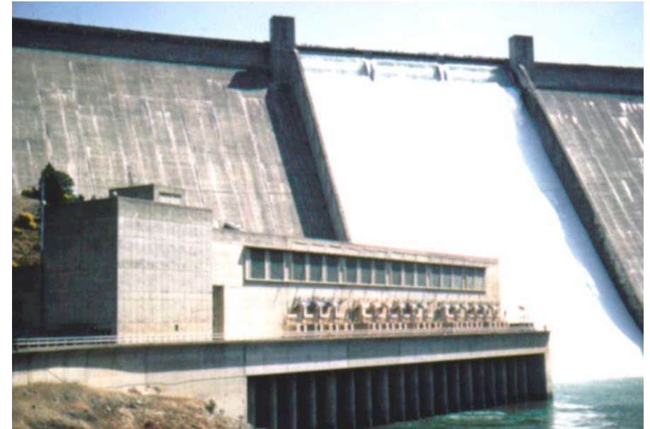
Powerplant at Shasta Dam
